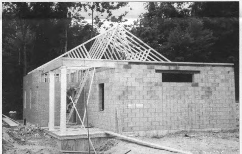
Building the new archives building. The main part of the building is a concrete bunker inside a decorative – and expendable – shell. Photograph by Betsey Harris, 1996
