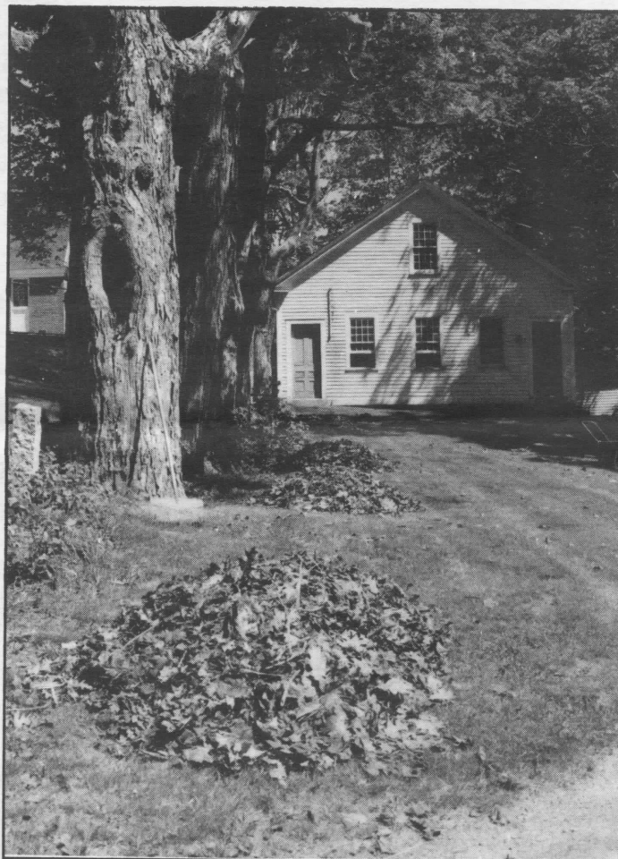
Years of leaves ready to be removed from the Schoolhouse yard.
